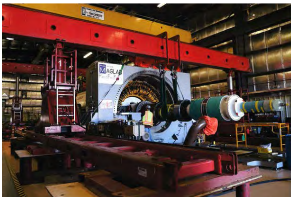
Figure 4.4.13: The rotor was removed from generator housing for further investigation and repair (September 2019).
