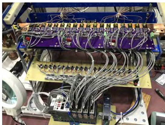
Figure 2.10: MOSFET bank testing setup.
